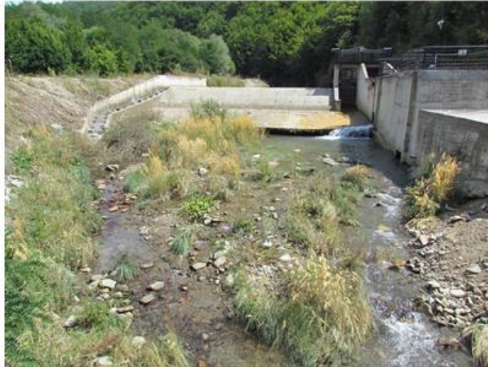
Figure 2. An example of RRHP installed at a montane stream in Serbia, with the common hydrological situation occurring at least during the eight months each year (left, the disfunctional, vertical-slot fish pass with the scarce, insufficient water flow; middle, the dam diverting the water to the pipeline; right, the concrete dam's overflow for the excessive water, ending with the pipeline's overflow outlet on the side cover of the pipeline's beginning; notify the surplus of water from the maximal installed amount of abstraction at the intake facility and pipeline, going back to the stream bed, while the fish pass remained without enough water) (personal photo library).
